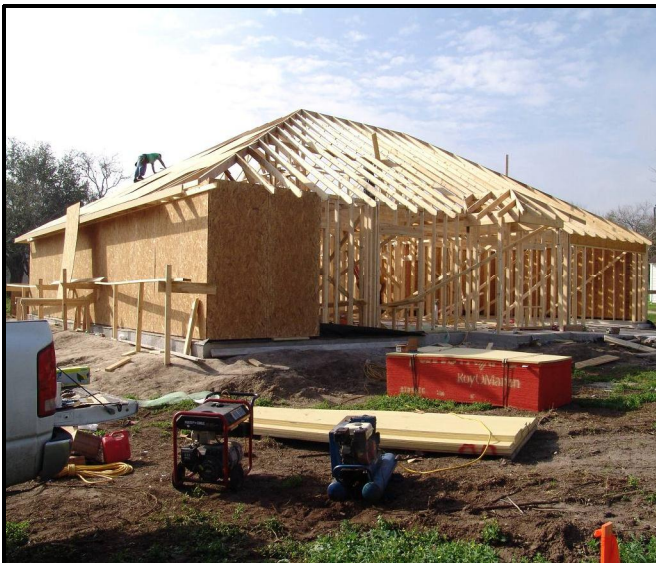
Construction begins on new IDD group home in Beeville.
